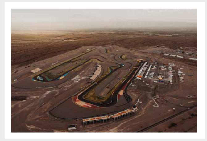
Located in the department of Albardón, the 4,254-meter layout has constant ups and downs along the route, artificially generated with a soil movement of more than 700,000 m3. It also has two alternative circuits of 3,500 and 2,500 meters in length.
